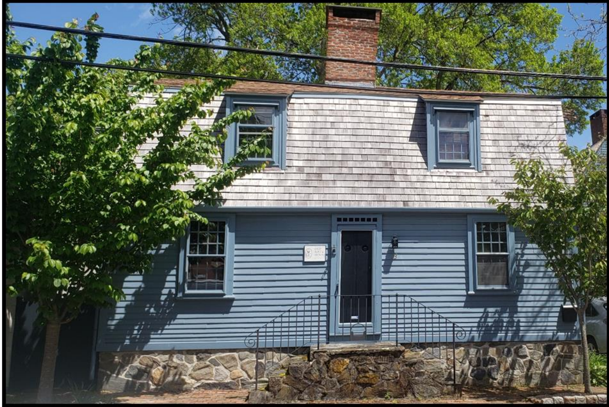
Figure 2:8 This gambrel roof, wood-framed dwelling was built in 1717 and was the home of Nathaniel Rodman – buried in God’s Little Acre. It was originally located on Warner St. but was moved during in the 1960’s during Newport’s redevelopment program. Today the dwelling is located on 13 Second Street. Image by Marjorie Drew, May 2019.
